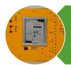
Synchronization relay to connect the generator to the grid.
