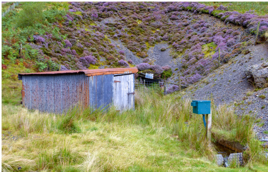
Outdoor View of Enclosures (Severn Trent Services, 2018)
