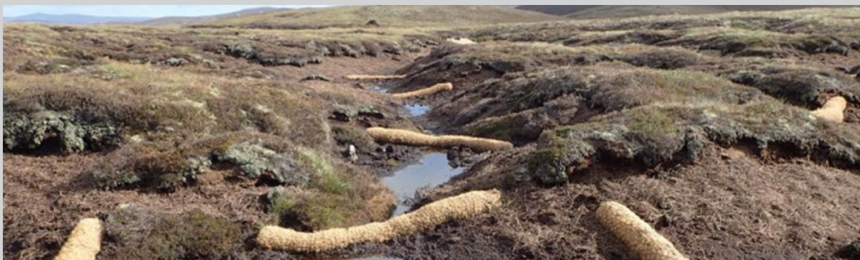
Peatland Restoration Using Coir (Coconut) Log Dams (Stephen Corcoran, 2018)
